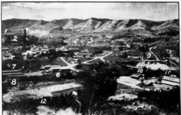
Panoramic view of operations in the Tavua Basin on Viti Levu Island.
